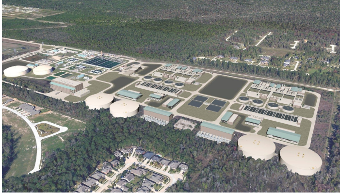
A water purification plant around Houston, Texas
